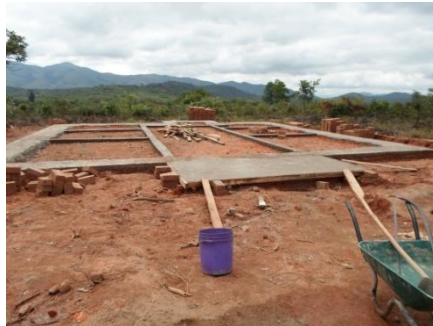
The foundation slab for the Health Post
