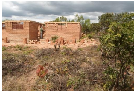
Health Post at ring beam Level
