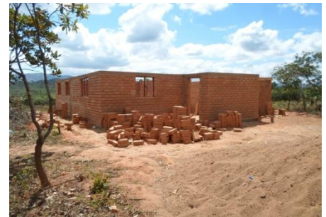
Health Post at ring beam Level
